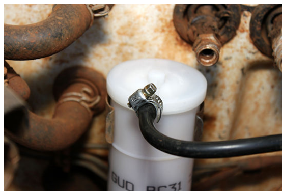
Fig: Photographs of Replacing Fuel Filter
